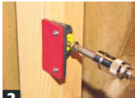
2 Click marker tool into Fix (bracket) to give position for button. Drill and fix button to frame with 5mm screw
